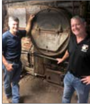
Bill and Todd Ray in front of the Mill's 1873 boiler.
